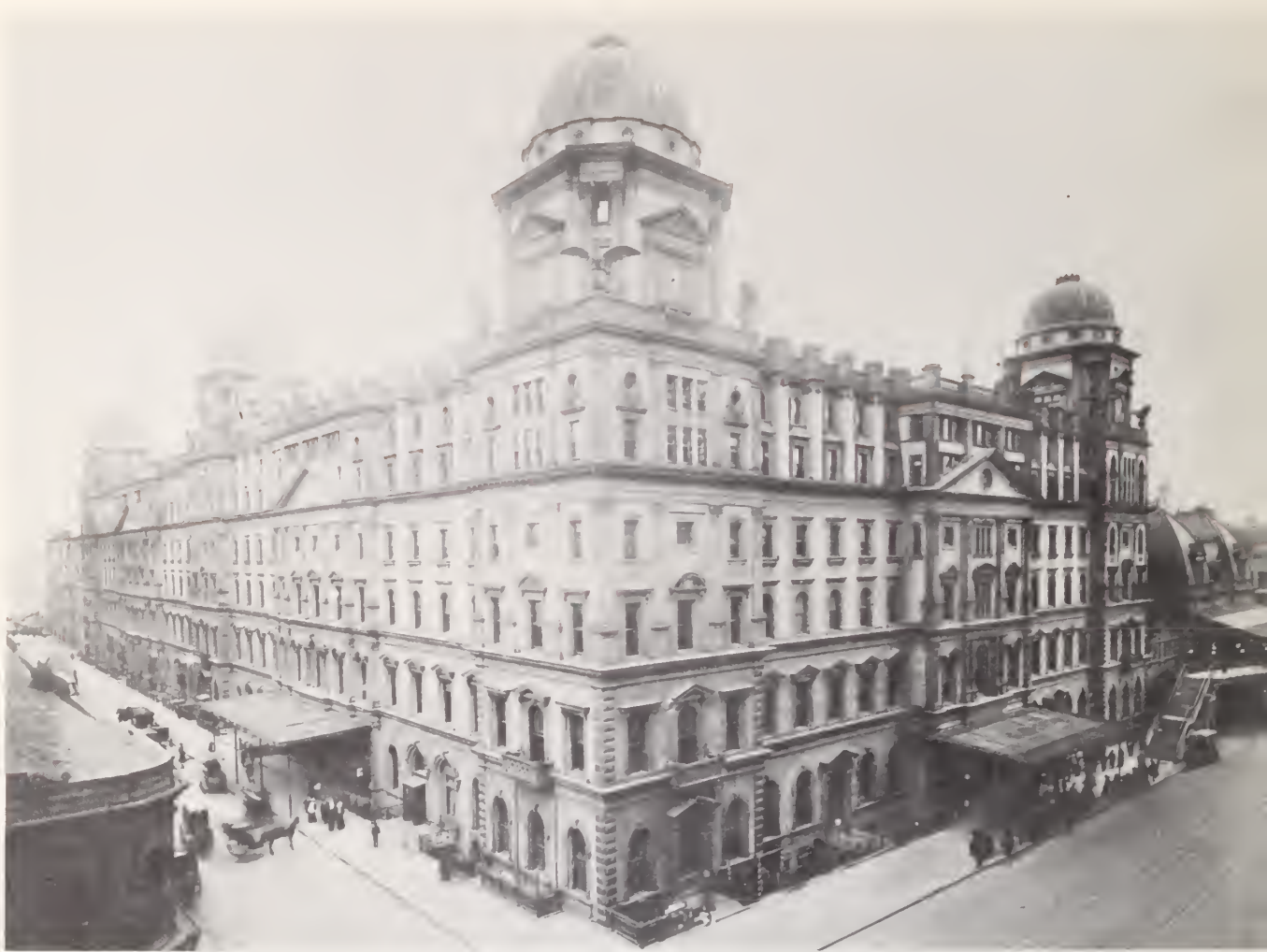
Fig. 10. Main facades, Grand Central Depot after the remodelling of 1900. The original mansard roofs were removed to make way for three additional floors. Exterior walls were resurfaced with rusticated stucco.
